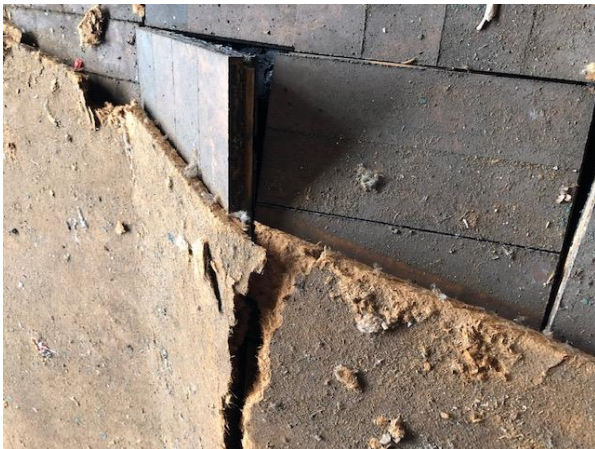
P-18 Fallen section of roof decking
