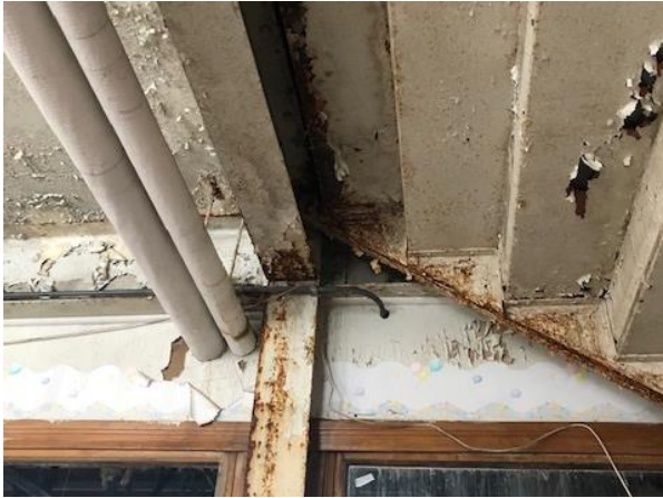
P-7 Corroded stair stringer and connection
