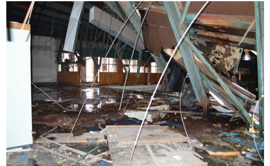
Roof collapse in the Main Drill Hill (Jefferson Avenue Block); scrappers removed bottom chord of roof truss
