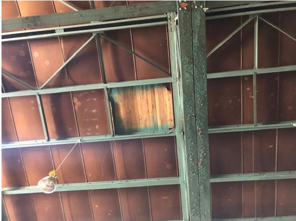
P-17 Deteriorated roof decking
