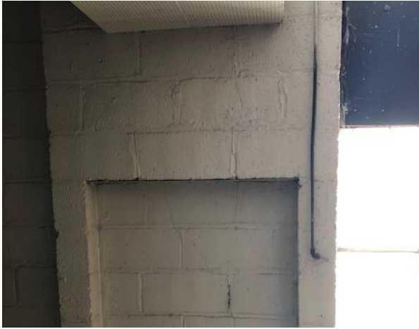
P-16 Hairline cracking at truss bearing pocket
