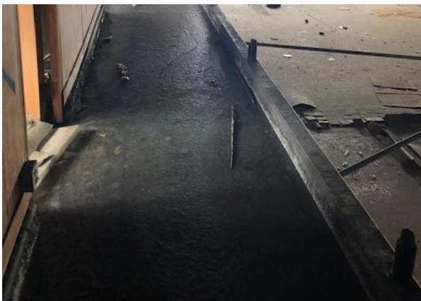
P-9 Missing guardrail
