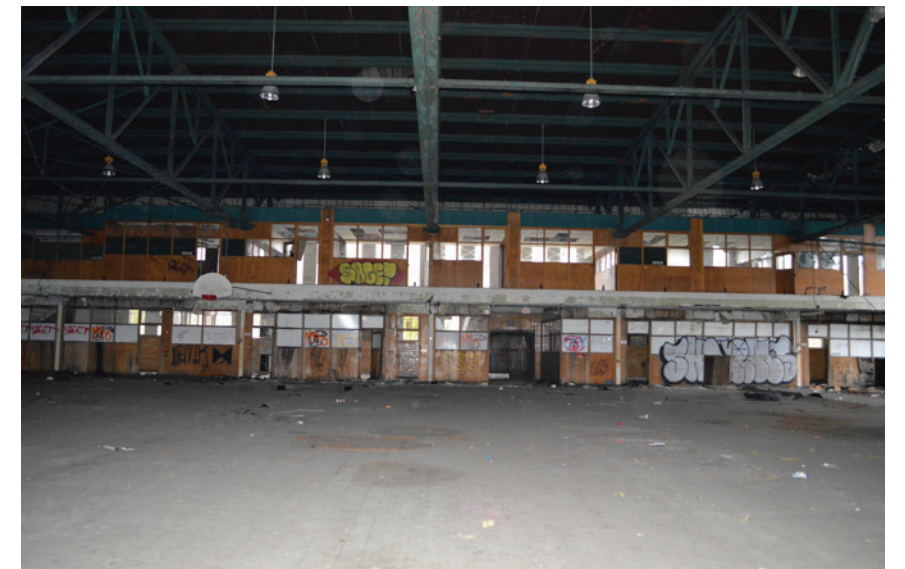
High-bay drill hall with exposed trusses
