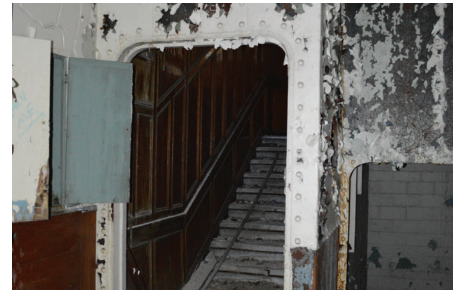
Reclaimed steel bulkhead from a mothballed ship
