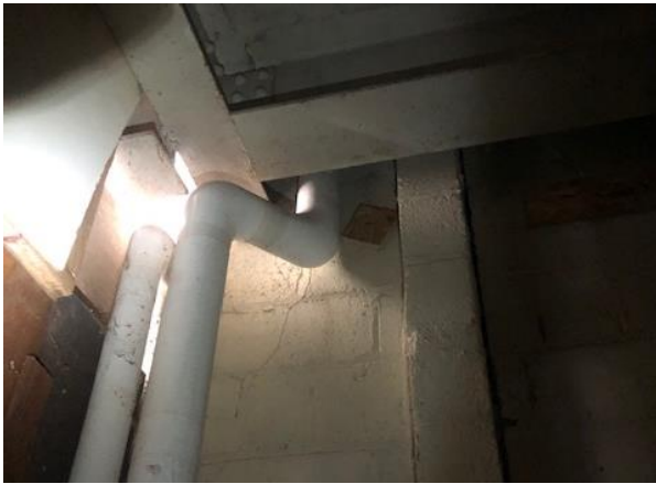
P-8 Masonry wall crack at bearing pocket
