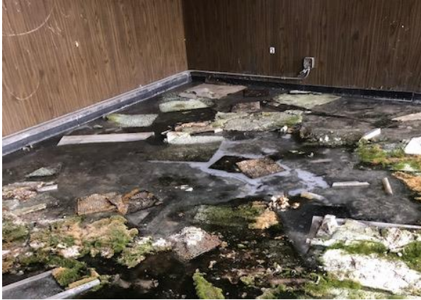
P-4 Mezzanine structural slab water ponding
