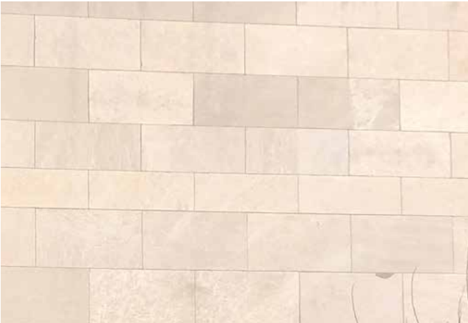
LIMESTONE PANELS FROM SOUTH BUILDING
