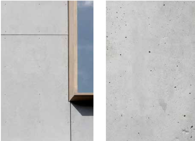
CAST-IN-PLACE ARCHITECTURAL CONCRETE FOUNDATION WALLS
