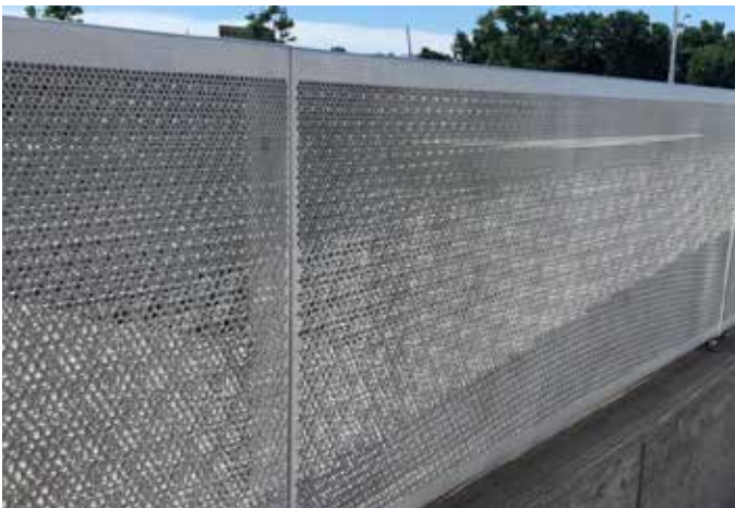
PERFORATED ALUMINUM GUARDRAIL
